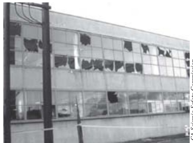
Figure 56 —The windows in this San Francisco building probably broke because its frame flexed too much in the Loma Prieta earthquake of 1989.
