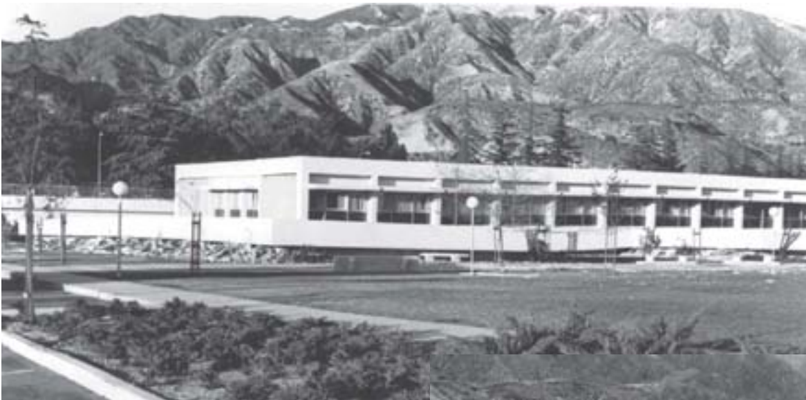
After the Earthquake
