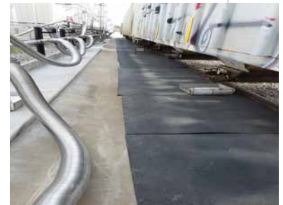
At Sonoco’s Chillicothe, Mo., facility, spillage is collected prior to entering storm drains using catch bins or rubber mats.
