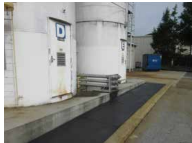
At Sonoco’s Chillicothe, Mo., facility, spillage is collected prior to entering storm drains using catch bins or rubber mats.
