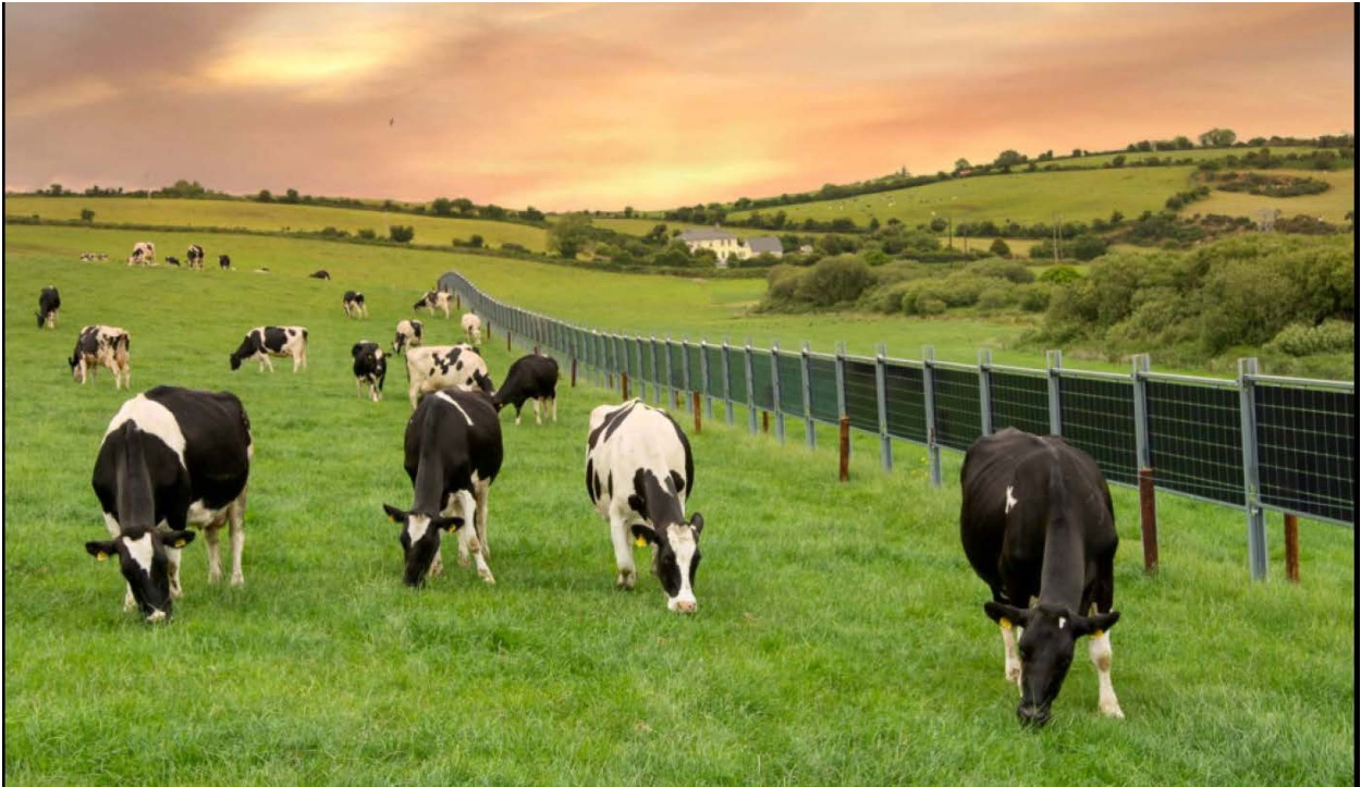
Figure S-9: Cattle grazing near vertical bifacial solar panels: Solar Farm Foran I (Ireland) Photo credit: Next2Sun GmbH, Germany, with permission
