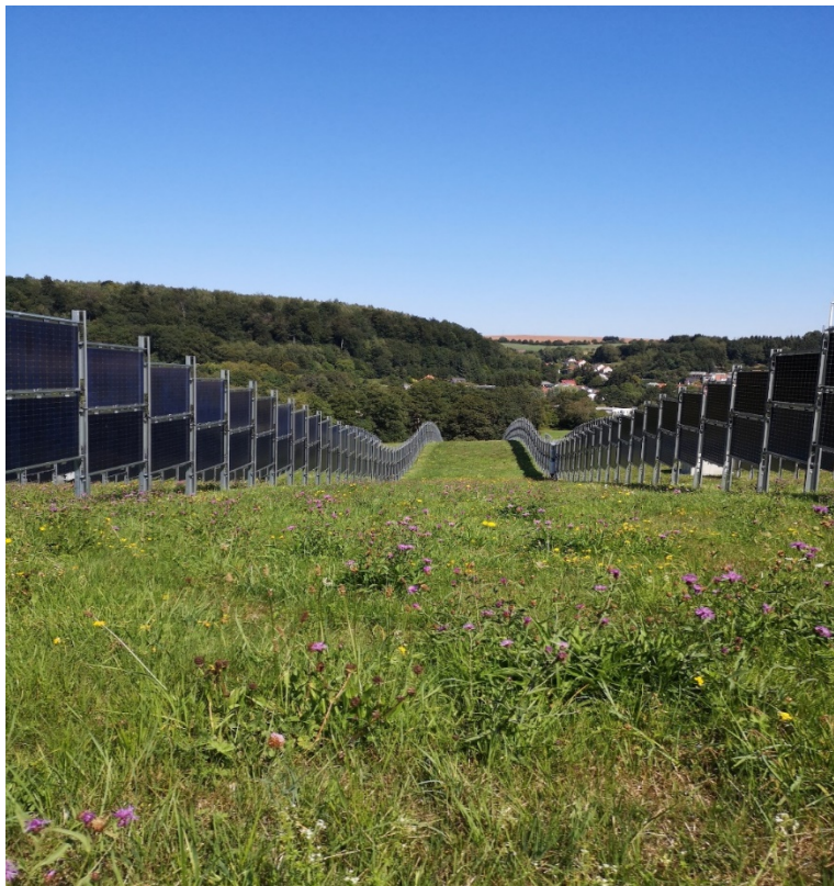
Figure II-4: Vertical, East-West solar panel configuration Photo Credit: Next2Sun, GmbH, with permission
