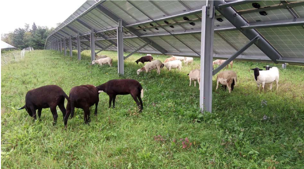
Figure II-1: A Ground mounted solar installation, showing small construction footprint; the panels also provide shade. Source: The American Solar Grazing Association ; with permission.
