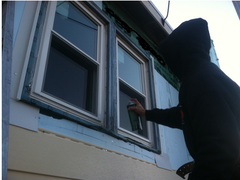
Figure 18. CBK WRB study air sealing demonstration
