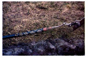
Coax-Cablecon can be plowed-in or laid in open trench if soil will not accept cable plow. Either way, continuous one-piece Coax-Cablecon beats hand work required with metal or PVC duct. If trench depth exceeds minimum bend radius of Coax-Cablecon, no sweeps or elbows are needed for easy, continuous duct termination. Transition fittings are available for joining to other systems.
