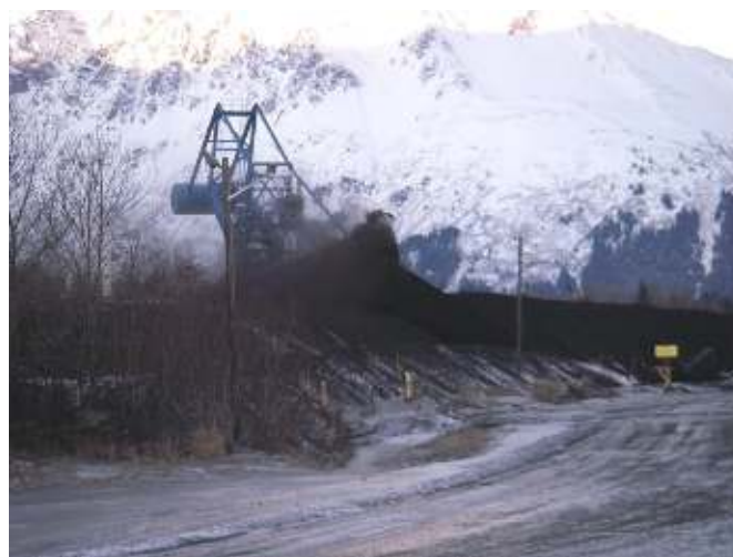
Coal dust from coal stockpiles blows in winter winds in Seward. Photo: Russ Maddox
