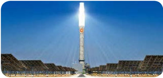
Gemasolar, Seville, Spain. Courtesy of www.torresolenergy.com
