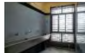
DRINKING WATER TROUGH
