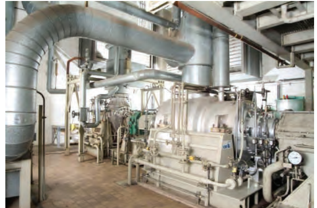
Boiler feed pump installed in : Pertamina, RU II, Balikpapan Cikarang Listrindo Power Plant
