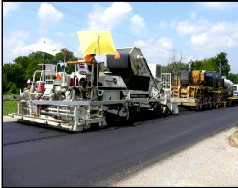
Figure 1-1: Cold In-Place Recycling (CIR) in field (Moore, 2013)
