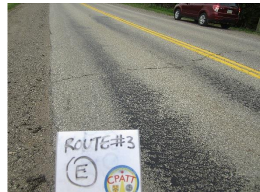
Asphalt Flushing
