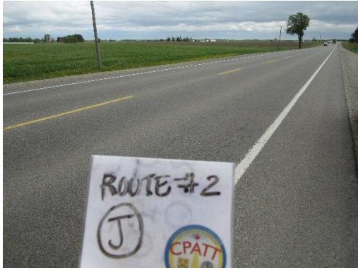
Minor to no thermal cracking
