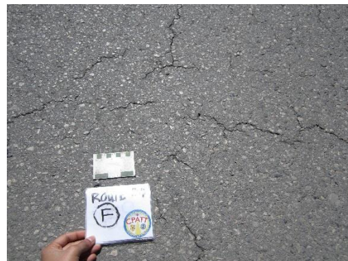
Micro cracking
