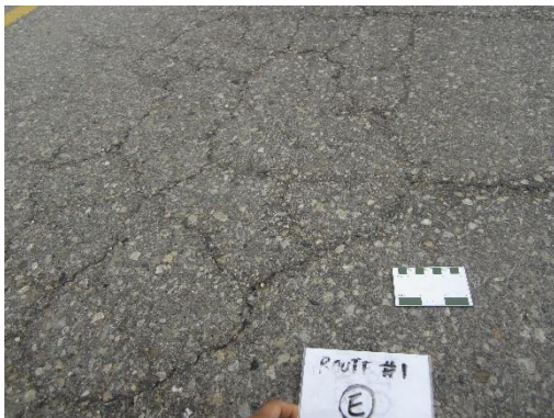
Alligator cracking
