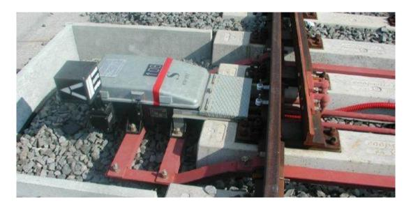
Figure 34 The photograph of P80 point machine installed near the track [23]
