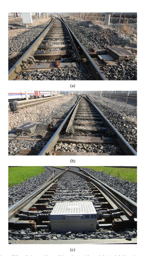
**Figure 12** Installation positions of the point machines: right (a), left (b) and central (c) [12]
