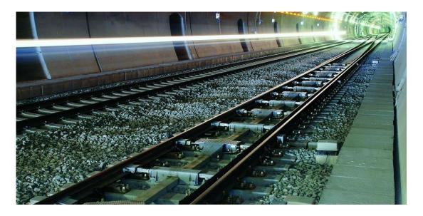
Figure 35 Hy-Drive point machine solution installed on a multiple drive turnout [24]
