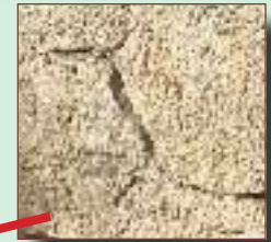
2000 YEAR-OLD EARTHQUAKE CRACK
