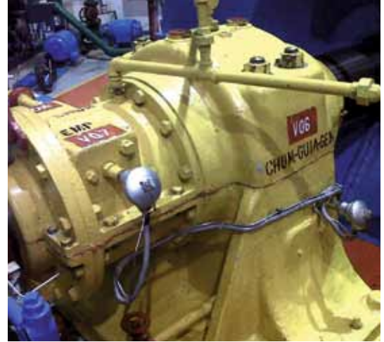
Bearing temperature measurement (vertical unit) CFE CH El Encanto, Veracruz, México
