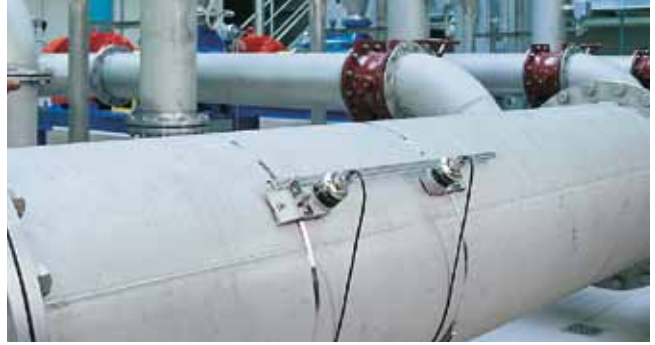
Clamp on ultrasonic flow measurement in the main pipe. CFE CH La Boquilla, Chihuahua México
