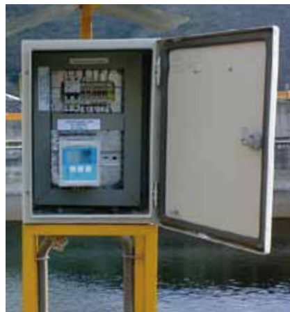
Dam ultrasonic time-of-flight level measurement with Prosonic S at CFE CH El Caracol, Guerrero, México
