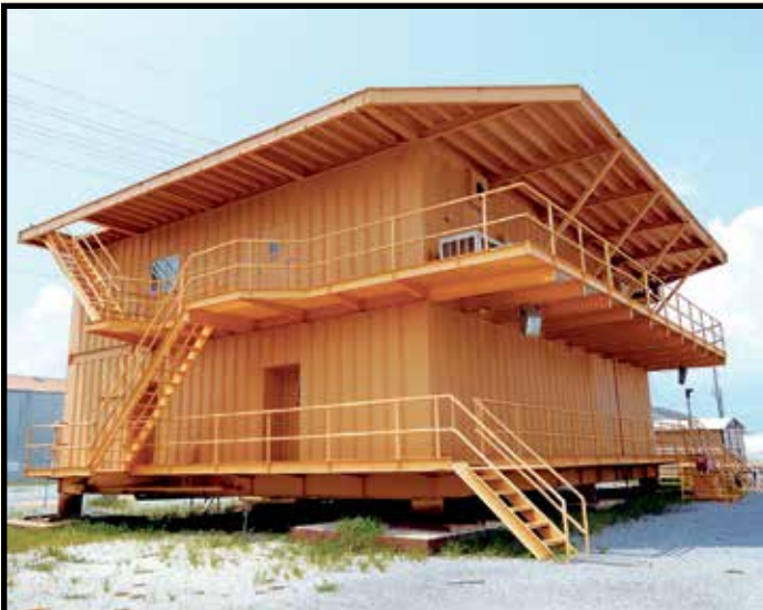
PORTABLE OFFICE BUILDING
