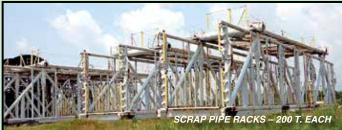
STRUCTURAL STEEL AND PIPE (DAY 5)
