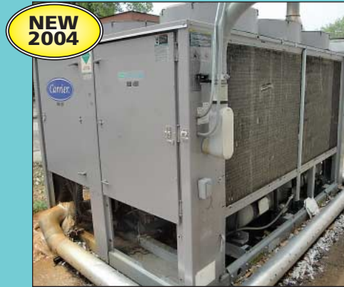
Carrier Model 30GXN106-A-661KA Packaged Skid Mounted Chiller System
