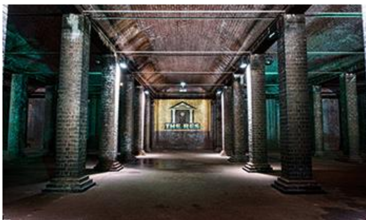
Figure 4-2: ‘The Res’ – a 19 th century underground drinking water reservoir located on The Hill
