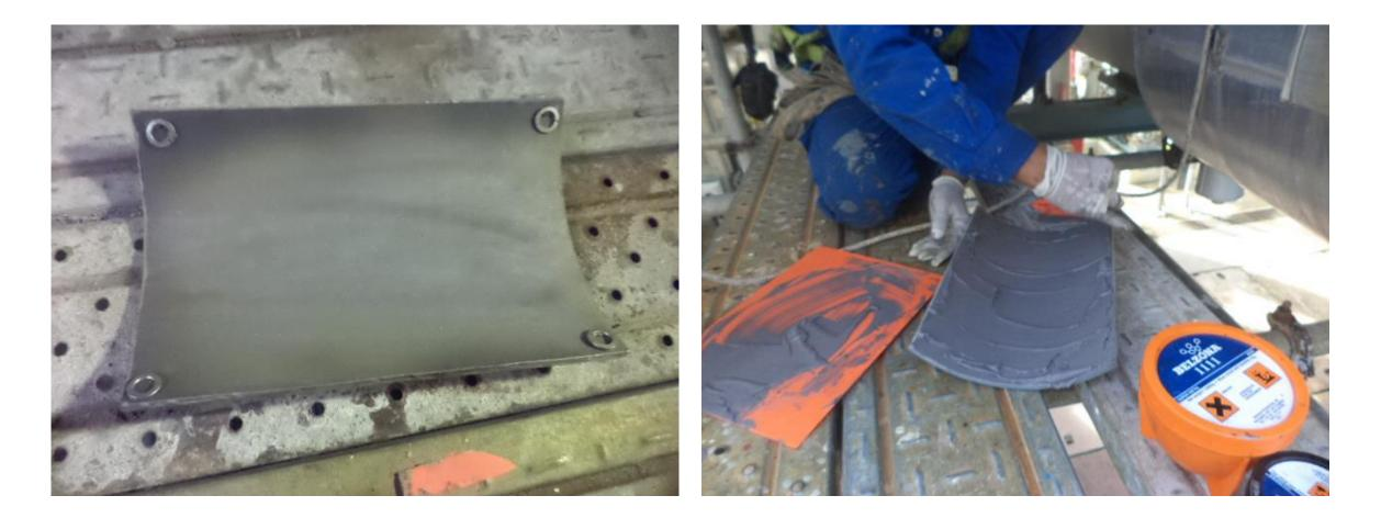
Apply Belzona 1111 on the metal plate
