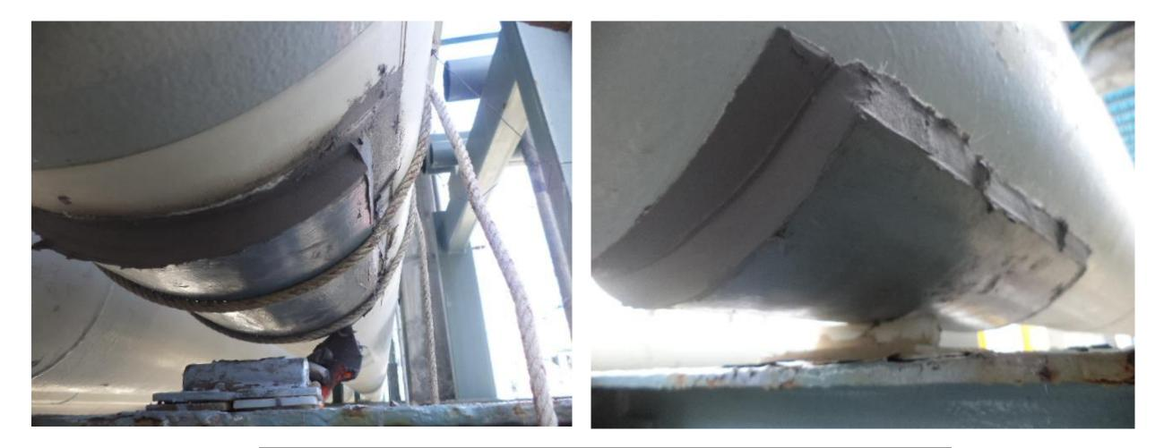
Bond metal plate with corroded pipe
