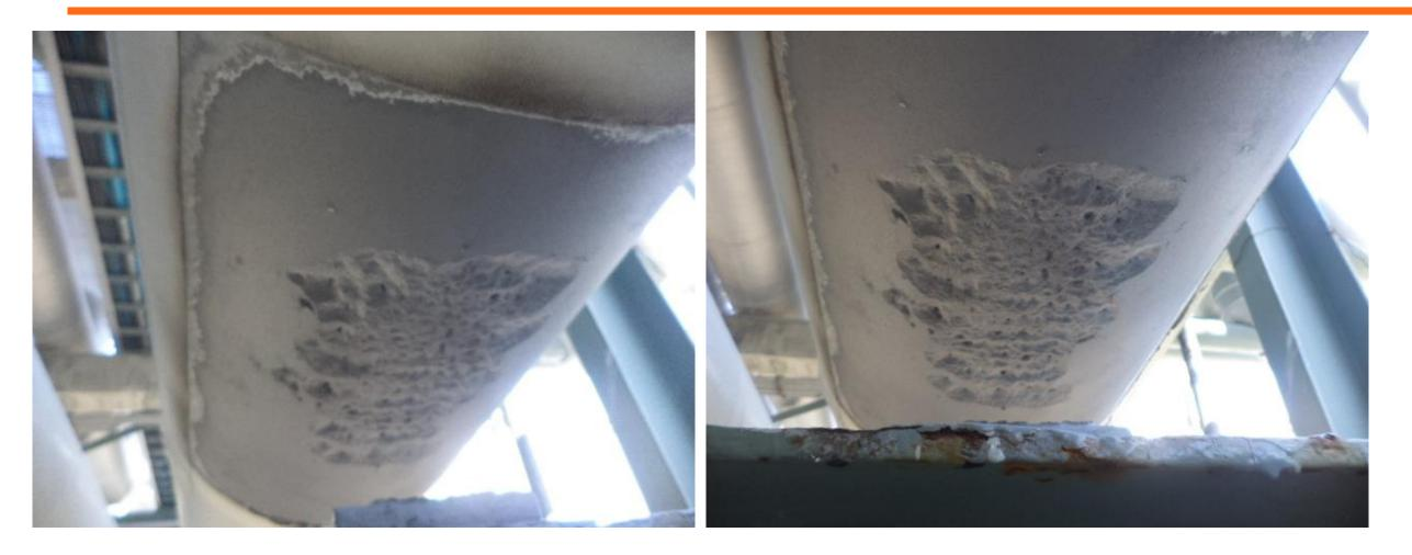
Condition of Corrosion Under Support – After Wet Blasting Severe metal loss revealed
