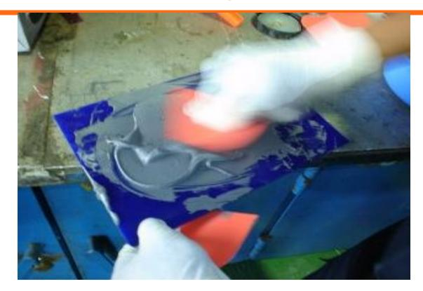
• Belzona 1111 was mixed and applied to the defect area
