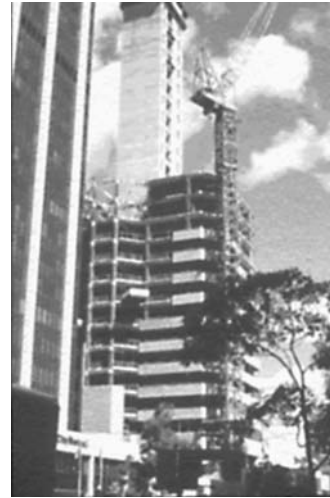
FIGURE 51.5 Composite construction, Forrest Place, Perth.
