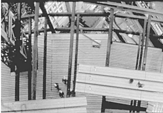
FIGURE 51.2 Composite steel–concrete floors, Grosvenor Place, Sydney.
