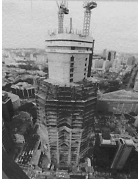
FIGURE 51.6 Composite construction, Republic Plaza, Singapore.
