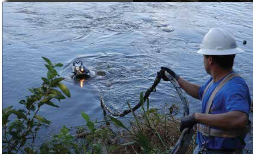
After free-flowing leak detection inspections are completed on large-diameter pipelines, the tools are retrieved and leak locations are recorded for repair and to determine sections with high failure rates.
