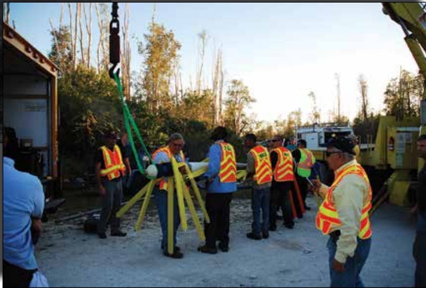
Nondestructive, free-flowing electromagnetic technology is used as part of an annual leak detection program that assesses pipes without shutting them down.
