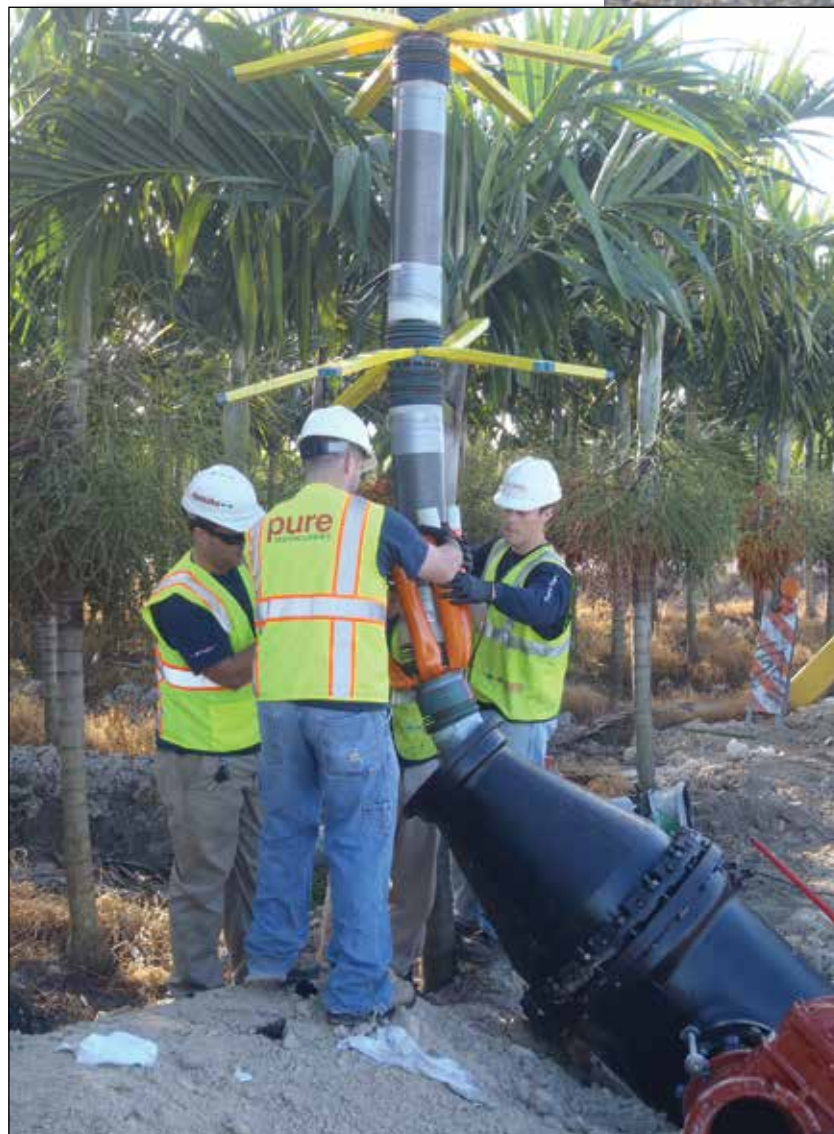
An electromagnetic tool is inserted into a live pipeline to identify prestressing wire breaks in one of Miami-Dade Water and Sewer Department’s prestressed concrete cylinder pipes.
