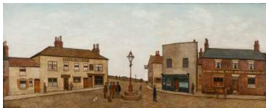
Bridge Foot, Castleford, Yorkshire Thomas Wainwright
