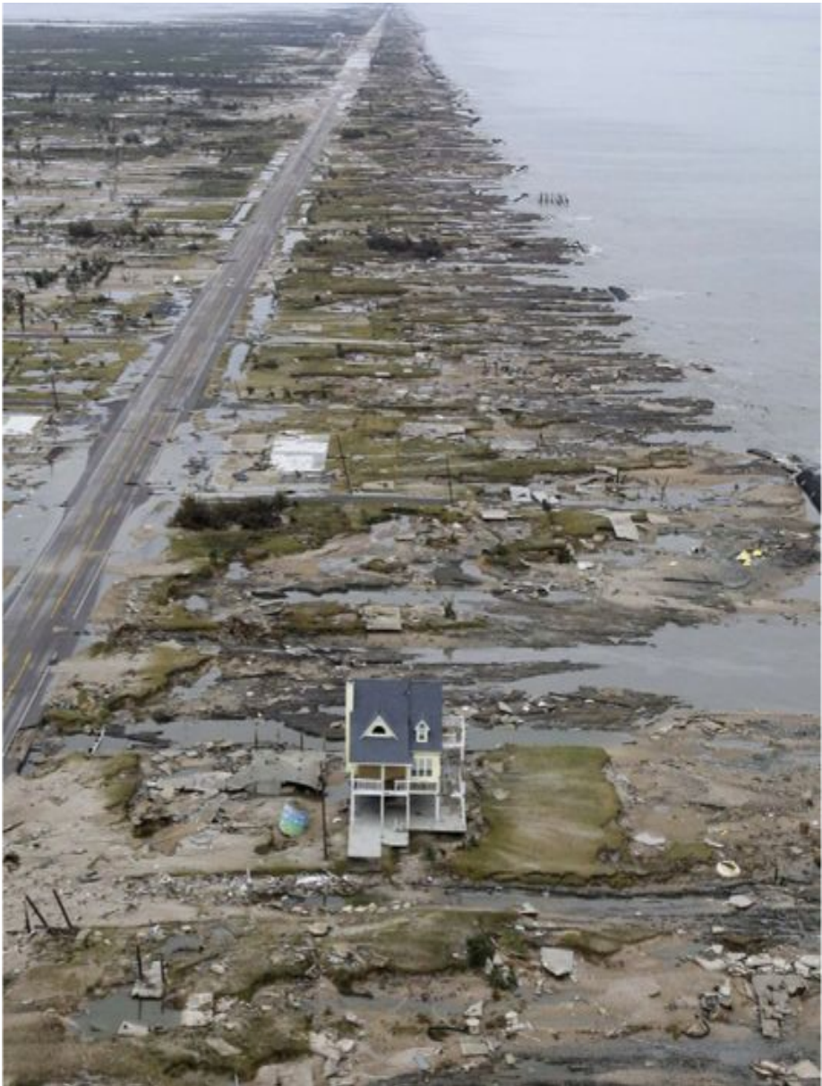
A picture of the coast near Gilchrist, Texas, after Hurricane Ike in 2008. This home's owners lost their previous home in Hurricane Rita in 2005. After Rita, they decided to build their new home to withstand a Category 5 hurricane. After Ike, it was the only coastal home left standing.
