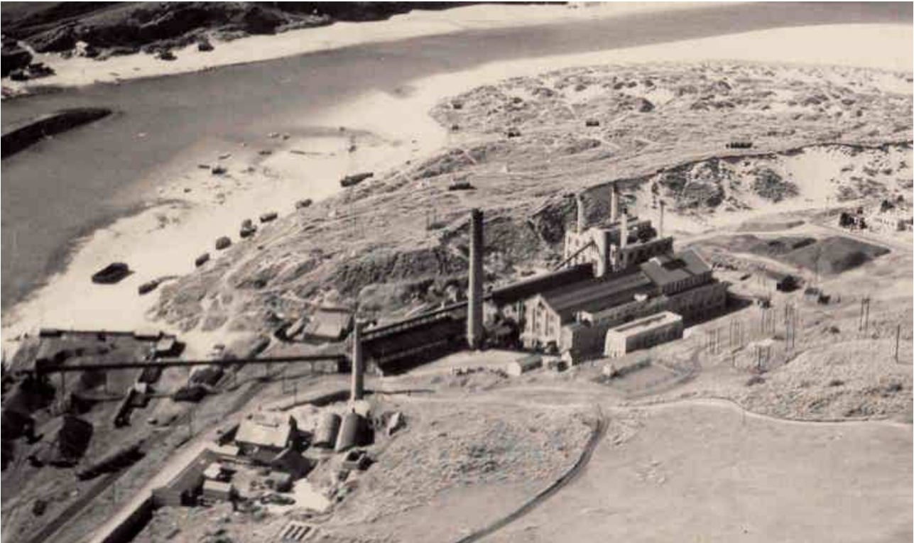
Figure 2: Hayle power station circa 1934.
