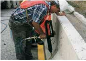
Anchoring a concrete traffic barrier wall to concrete bridge deck.
