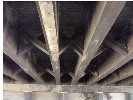
Photo 11: Bridge I-13-G – Repaired Girders Source: CDOT
