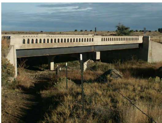
Photo 21: Bridge M-21-B Source: CDOT
