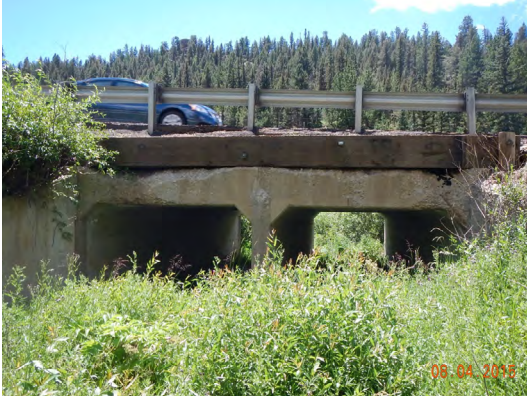
Photo 15: Bridge I-15-T Source: CDOT
