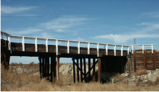
Photo 36: Bridge N-21-C Source: CDOT
