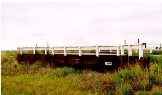
Photo 33: Bridge M-22-Y Source: CDOT
