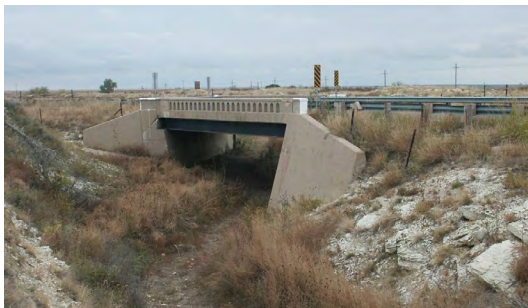
Photo 30: Bridge M-22-U Source: CDOT
