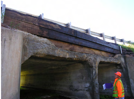
Photo 13: Bridge I-15-AO – Timber Planks Retaining Roadway Source: CDOT
