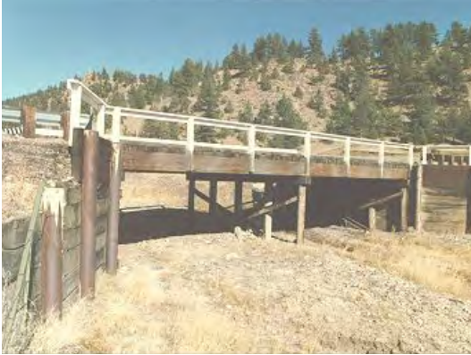
Photo 4: Bridge J-14-C Source: CDOT
