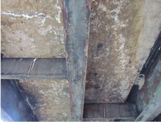
Photo 31: Bridge M-22-U – Typical Deck Condition Source: CDOT
