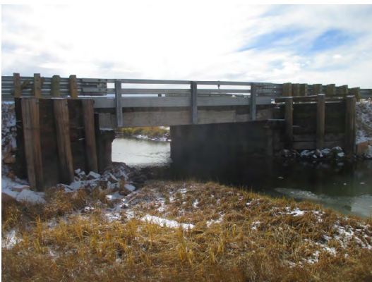
Photo 18: Bridge H-13-N Source: CDOT
