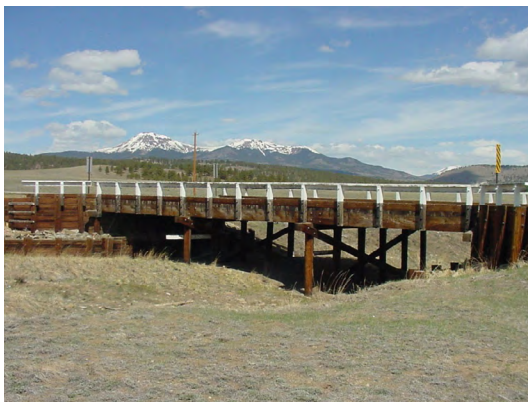
Photo 10: Bridge I-13-G Source: CDOT
