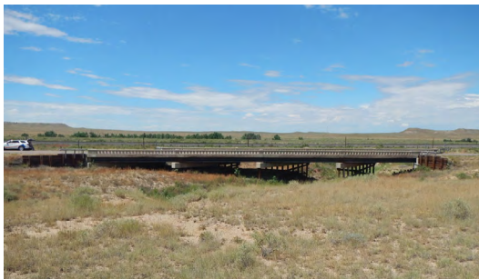
Photo 39: Bridge N-21-F Source: CDOT
