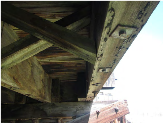
Photo 28: Bridge M-21-J – Repaired Girders (Typical) Source: CDOT
