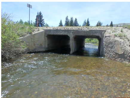
Photo 1: Bridge G-12-C Source: CDOT
