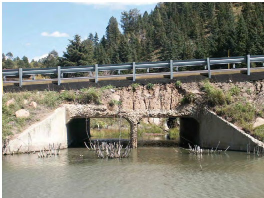
Photo 12: Bridge I-15-AO Source: CDOT
