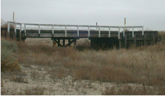
Photo 27: Bridge M-21-J Source: CDOT
