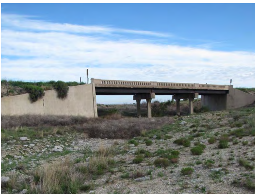
Photo 24: Bridge M-21-C Source: CDOT
