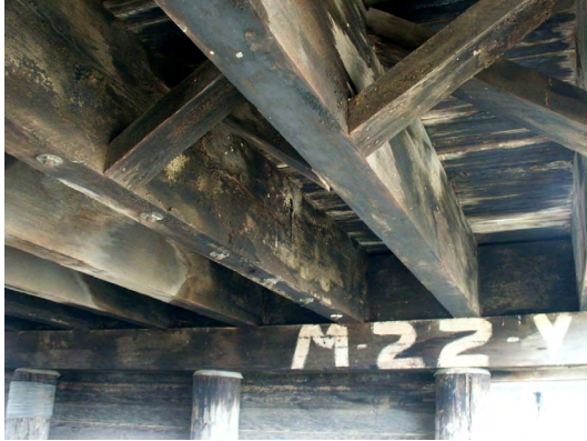
Photo 34: Bridge M-22-Y – Repaired Girders Source: CDOT
