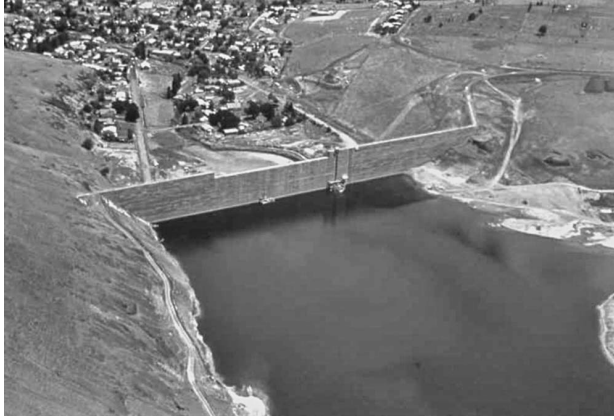
FIGURE 20.2 Willow Creek Dam in Colorado, which was the world's first major all RCC dam and used mostly 80 lb of cement and 32 lb of ash per cubic yard. (Photograph courtesy of Ernest K. Schrader.)
