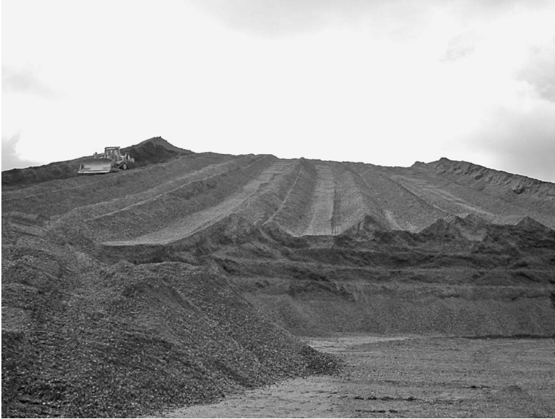
FIGURE 20.48 A large “all-in” aggregate stockpile with no segregation at Burnett Dam.
