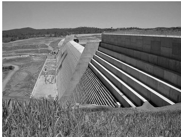
FIGURE 20.6 Burnett River (Paradise) Dam in Australia, which used 106 lb of cement per cubic yard (no ash). (Photograph courtesy of Ernest K. Schrader.)
