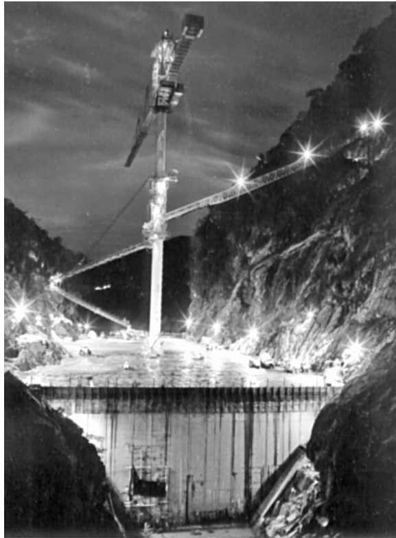
FIGURE 20.49 Tower belt with 320-ft reach at Miel I dam in Colombia.
