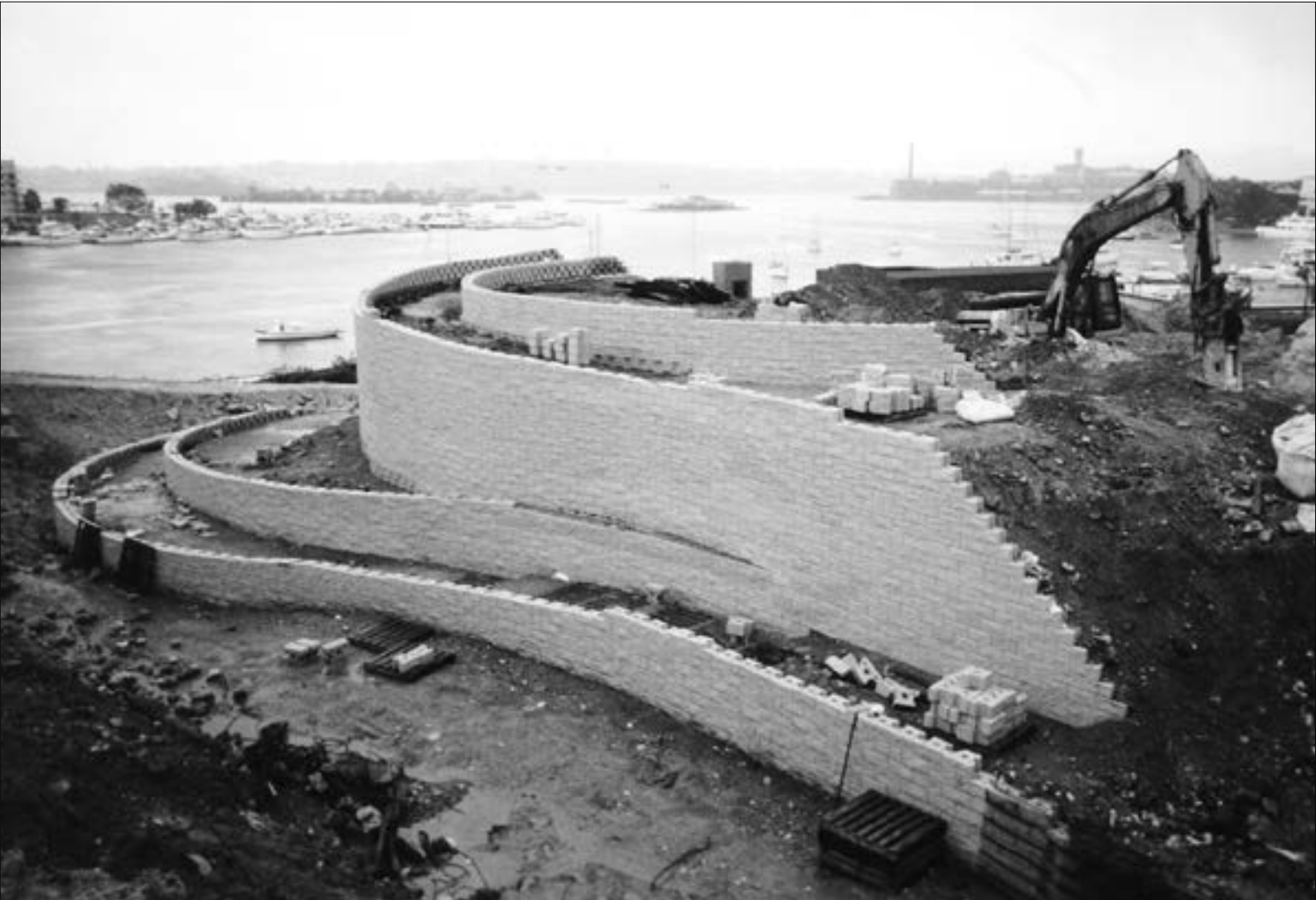
Balmain Foreshore Redevelopment, Sydney, Under Construction
