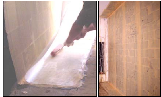
Fig. 10. R10 – Polyurea trowel-on & thermoplastic film.
