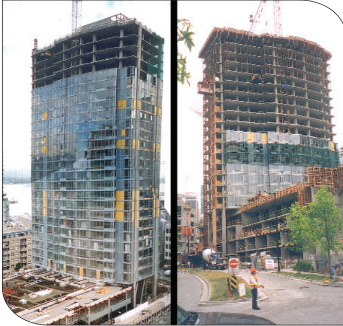
Figure 26. Bayview high-rise apartment. (Courtesy Ecosmart Foundation)
