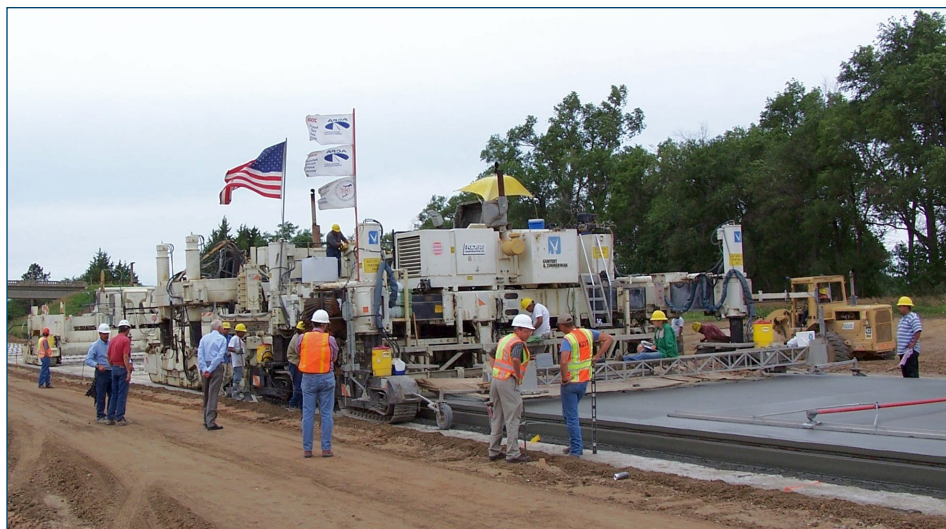
Concrete pavement placement
