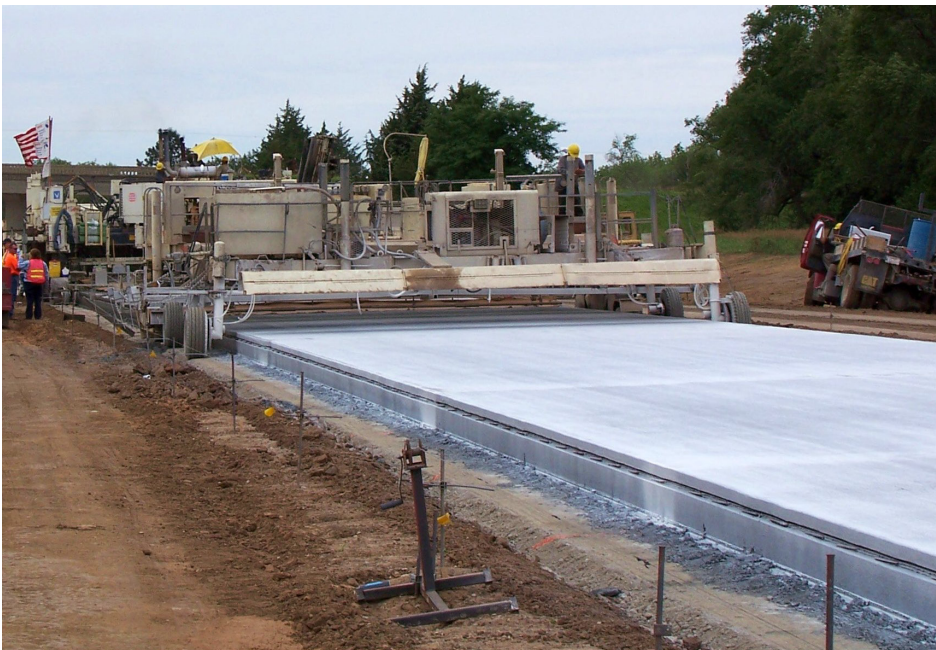
Pavement with cure applied
