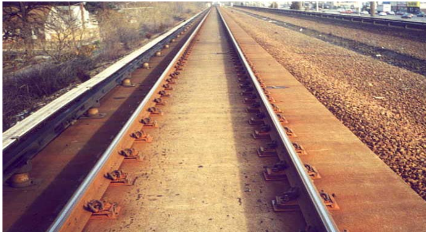
Figure 14 – The LIRR Messapequa Slab Track Section after 20 years of service
