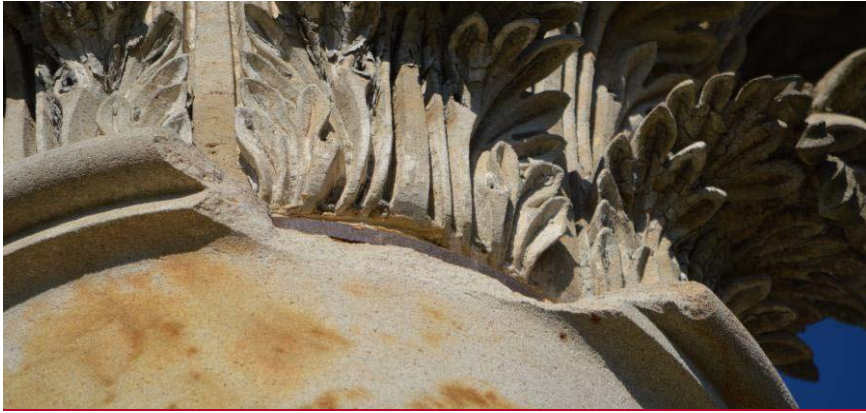
Figure 7: Detail of stone loss from L13's astragal, revealing its iron ring directly below the bottom edge of the capital.
