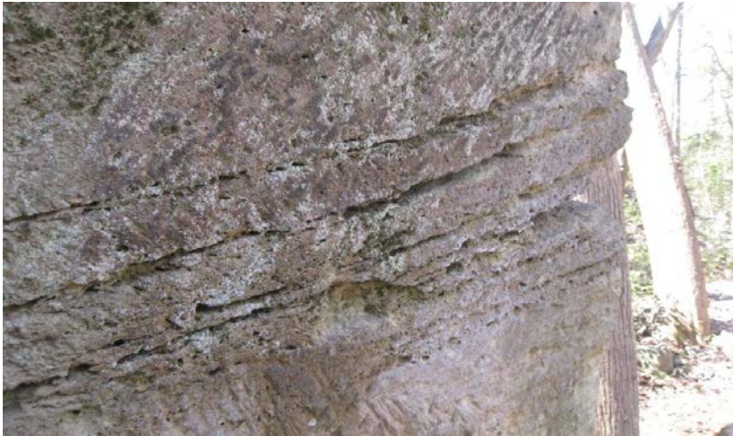
Figure 2: Quarry face on Government Island, a state park where Aquia Creek sandstone was once quarried, with horizontal voids indicating stone unsuitable for buildings (2013).
