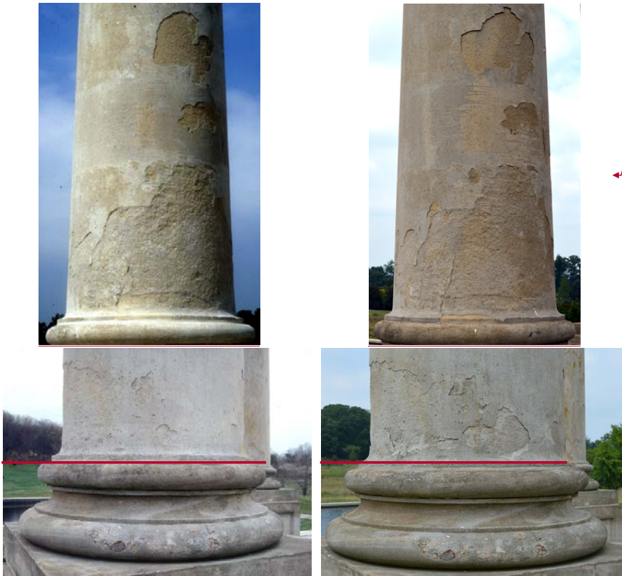
Figure 5. Contour losses on column L53 in 1988/2000 (Grissom).
