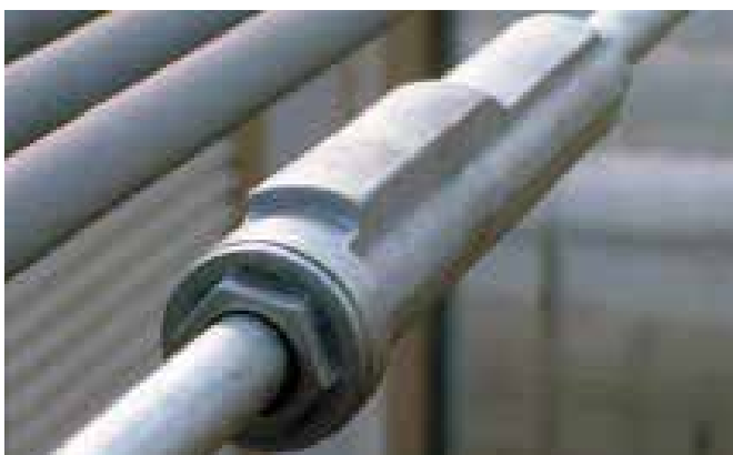
Figure 14A: Expansion fitting.
