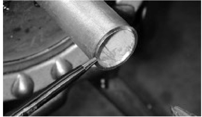
Figure 8: A minimal amount of pressure will remove the burr completely and eliminated possible flaring of the conduit end.
