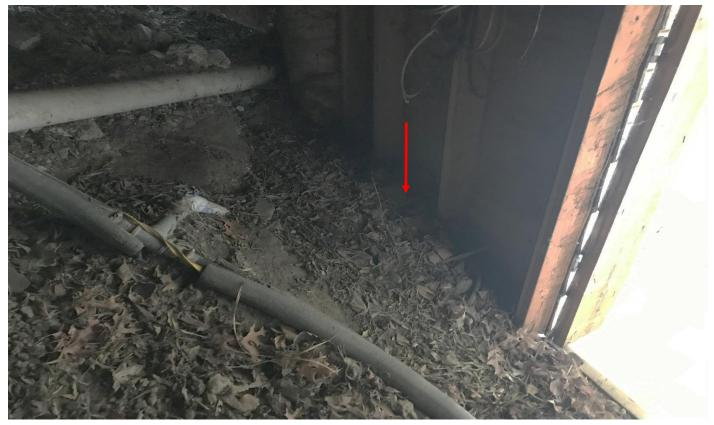
INCREASE EARTH TO WOOD SEPARATION AT THE CRAWLSPACE AREA BELOW THE GARAGE. ANY DECAYED OR DAMAGED MATERIAL THAT IS LOCATED AFTER THE AREA IS RE-GRADED MUST BE REPLACED AS IS FOUND TO BE REQUIRED.
