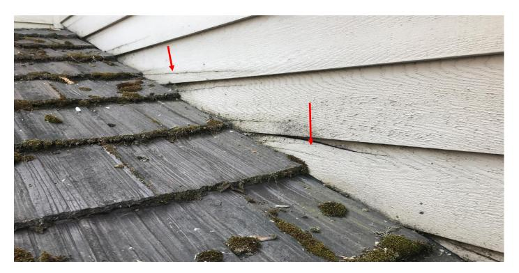
LOCATE AND REPLACE ANY DAMAGED SIDING MATERIAL ABOVE THE FRONT PORCH AREA. ANY DAMAGE THAT IS REVEALED AFTER THE SIDING IS REMOVED MUST ALSO BE REPLACED.
