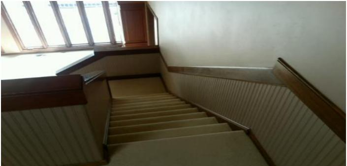
INSTALL A PROPER HAND RAILING ON THE INTERIOR STAIRWELLS.
