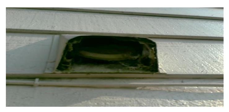
THE CLOTHES DRYER VENT AND PIPE IS CLOGGED WITH LINT AND IS A FIRE HAZARD. THE DRYER VENT LINE MUST BE PROFESSIONALLY CLEANED AND INSPECTED TO ENSURE IT IS SAFE AND IN PROPER OPERATING CONDITION.
