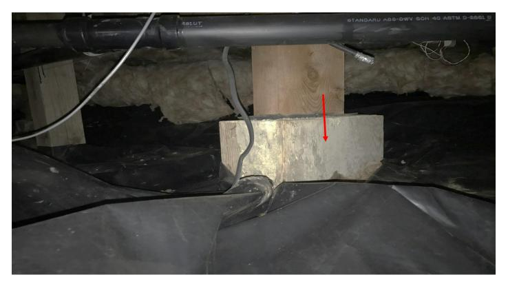
REMOVE ALL CELLULOSE DEBRIS FROM THE CRAWL SPACE AREA. CELLULOSE DEBRIS INCLUDE ALL WOOD, CARDBOARD, WOOD FORM TIES AND ANY OTHER FOOD SOURCE FOR WOOD FUNGUS GROWTH.
