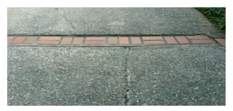
PREVIOUS SETTLING WAS NOTED AT THE DRIVEWAY. REPAIR ALL TRIP HAZARDS, SEAL ALL CRACKS AND ENSURE ALL RUNOFF IS PROPERLY ROUTED AWAY FROM THE STRUCTURE.
