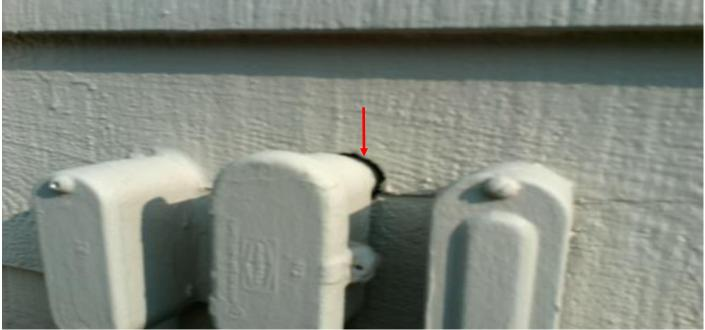
RE-CAULK ALL FAILING CAULKING AS LOCATED AT THE SIDING BUTT ENDS, TRIM WORK, CORNER BOARDS, WINDOW SYSTEMS AND AS FOUND TO BE REQUIRED TO PREVENT WATER MIGRATION INTO THE SIDING MATERIAL AT ALL SIDES OF THE HOUSE.
