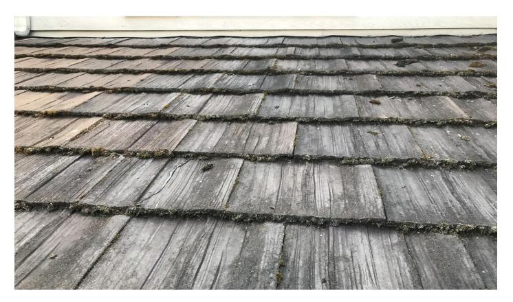
CLEAN THE ROOF WITH A METHOD THAT WILL NOT DAMAGE THE ROOFING SYSTEM, THE CLEANING MUST REMOVE ALL LICHEN GROWTH, MOSS, AND WIND BLOWN DEBRIS, AND IF ANY DAMAGED ROOFING MATERIAL IS LOCATED DURING OR AFTER THE CLEANING IT MUST BE REPLACED AS FOUND TO BE REQUIRED TO ENSURE THERE ARE NO ACTIVE LEAKS. THE GUTTERS AND DOWNSPOUTS AND TIGHT LINES MUST ALSO BE CLEANED AND ANY REPAIRS NEEDED MUST BE COMPLETED TO ENSURE THE SYSTEM IS PROPERLY DIRECTING ALL ROOF RUN OFF AWAY FROM THE STRUCTURE.
