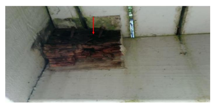
LOCATE AND REPLACE ANY AND ALL DAMAGED AND OR DECAYED DECKING, JOIST, FASCIA, RAIL BLOCKING AND STRUCTURAL MATERIAL AT ALL DECKS. ALL DAMAGED MATERIAL THAT IS UNCOVERED MUST ALSO BE REPLACED AS FOUND TO BE REQUIRED.
