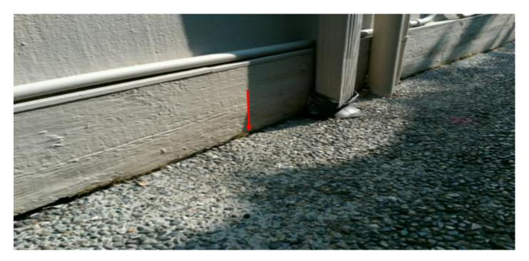
LOCATE AND REPLACE ANY DAMAGED AND OR DECAYED SIDING TRIM MATERIAL AT THE BOTTOM TRIM AT THE SOUTH SIDE OF THE HOUSE. ANY FURTHER DAMAGE THAT IS REVEALED AFTER THE SIDING IS REMOVED MUST ALSO BE REPLACED.
