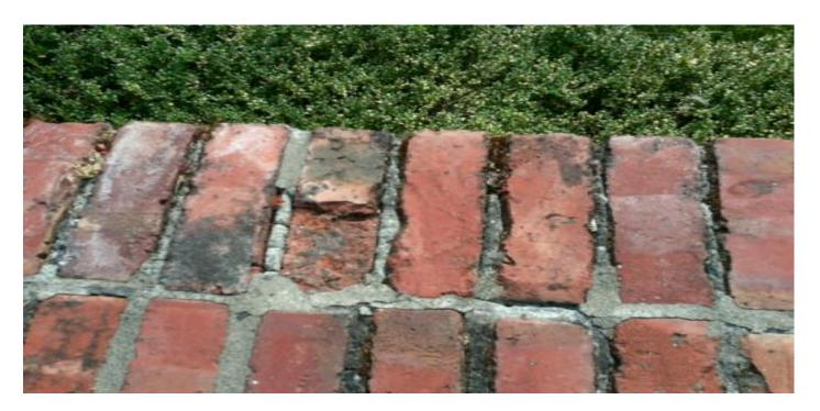
TUCK POINT THE BRICK WALL AT THE LOWER REAR DECK AS REQUIRED TO SECURE ALL BRICKS AND STOP FURTHER WATER DAMAGE.
