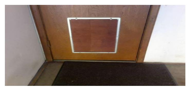
A PET DOOR HAS BEEN INSTALLED AT THE SOUTH GARAGE MAN DOOR. COMPLETE ALL REPAIRS AS FOUND TO BE REQUIRED TO RESTORE THE FIRE RATING TO THE DOOR SYSTEM.
