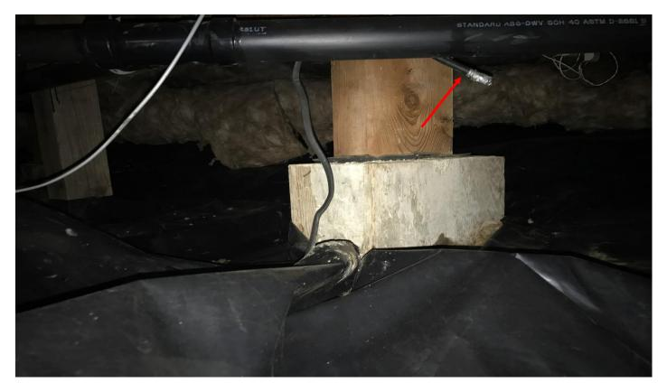
THE ELECTRICAL SERVICE MUST BE INSPECTED BY A LICENSED ELECTRICAL CONTRACTOR AND ALL REPAIRS FOUND TO BE REQUIRED MUST BE COMPLETED. THE REPAIRS MUST INCLUDE BUT NOT BE LIMITED TO: REPLACING ALL BREAKERS WITH TEXTURE OVERSPRAY AND INSPECTING THE PANELS TO ENSURE IT IS CLEAN OF ALL FOREIGN MATERIAL AND SAFE FOR USE, INSTALLING ALL LOOSE/EXPOSED WIRING IN THE CRAWLSPACE IN A JUNCTION BOX WITH A COVER PLATE AND ANY OTHER REPAIRS DEEMED TO BE REQUIRED AND OR LISTED WITHIN THIS REPORT.
