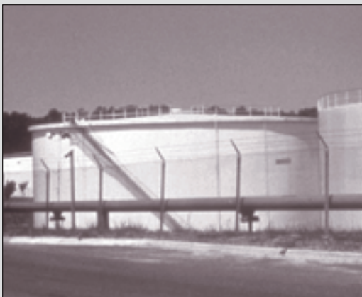
Chemical storage tank
