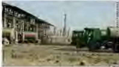
The Baiji oil refinery, north of Baghdad, is Iraq's largest fuel facility, producing 140,000 barrels a day.
