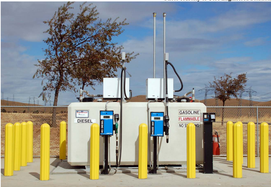
Figure 2 Dual Compartment Convault Protected AST (U.L. 2085)
