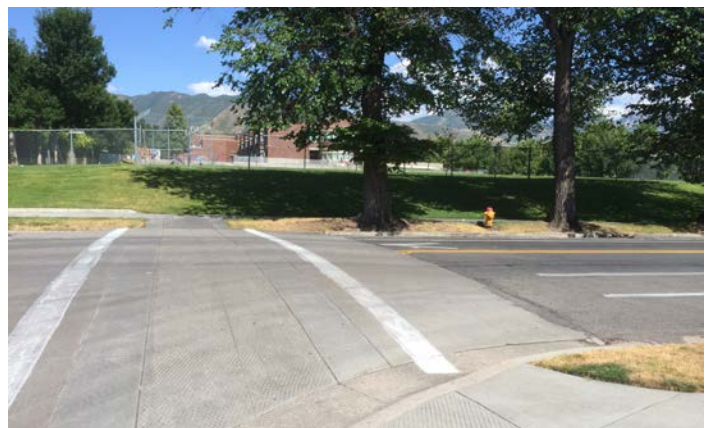
Raised crossings, such as this one near Uintah Elementary, are one traffic calming element that can make routes to school safer.
