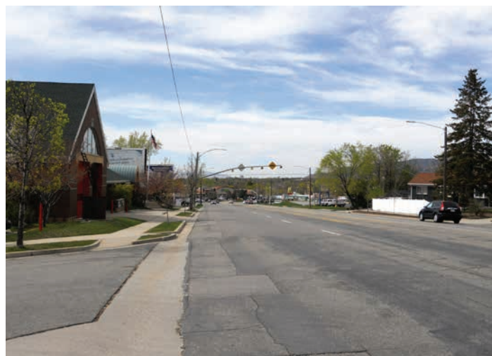
Foothill Drive and Parley's Way (shown above) are major corridors and should be designed to move people efficiently and safely.
