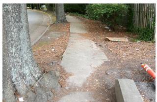
POOR SIDEWALK - PARKS AVE SIDEWALK IS LESS THAN 5'WIDE, CONTAINS FAILING PAVEMENT AND DOES NOT MEET AMERICAN DISABILITY ACT (ADA) STANDARDS
