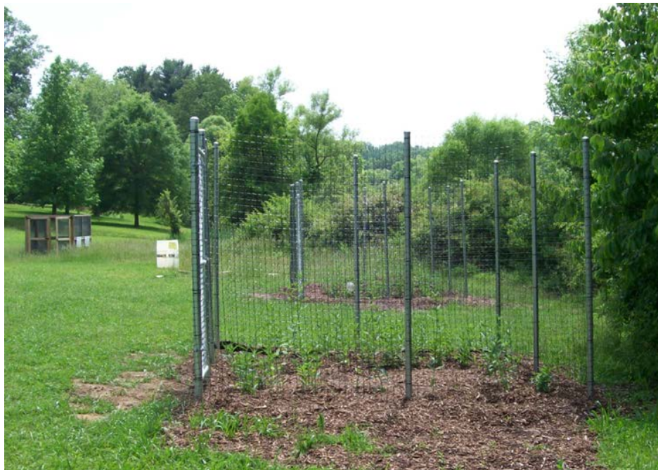
Welded wire deer fence, 10' x 10' x 8' high, with metal stakes and an open top. Photo by Ruth Eisenhour, Harford Glen Environmental Education Center.
