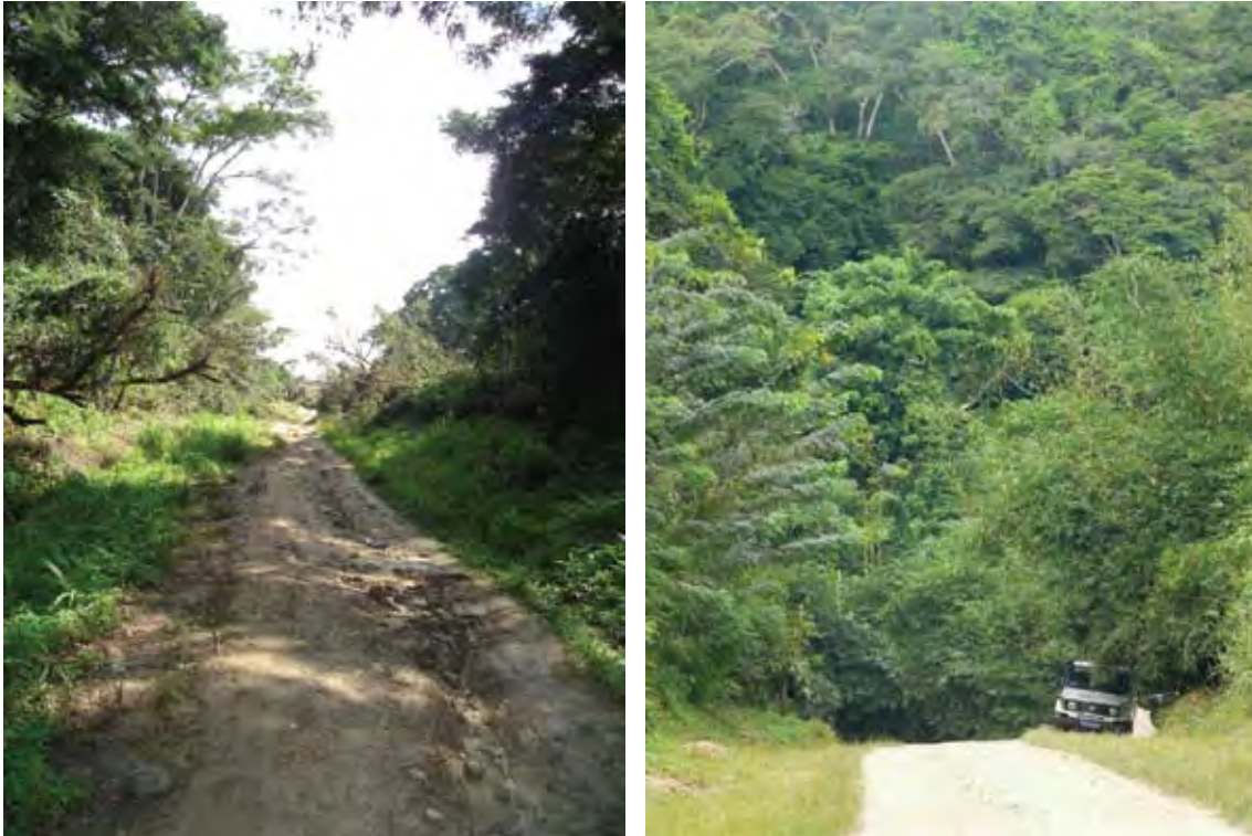
Figure 10. The Mbau-Kamango road (a) before rehabilitation in 2005 (© SODERU) and (b) after rehabilitation in 2008 (© ZSL)
