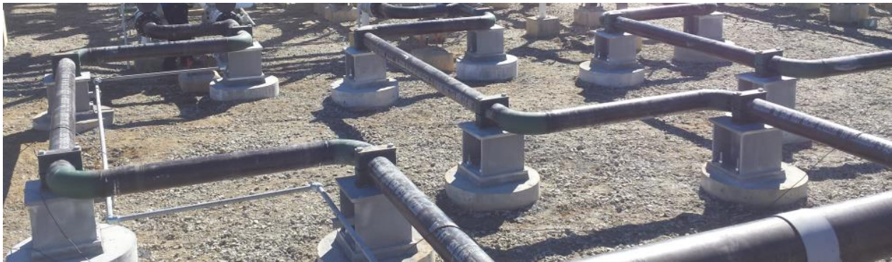
Figure 3. Examples of support location with thermal flexibility
