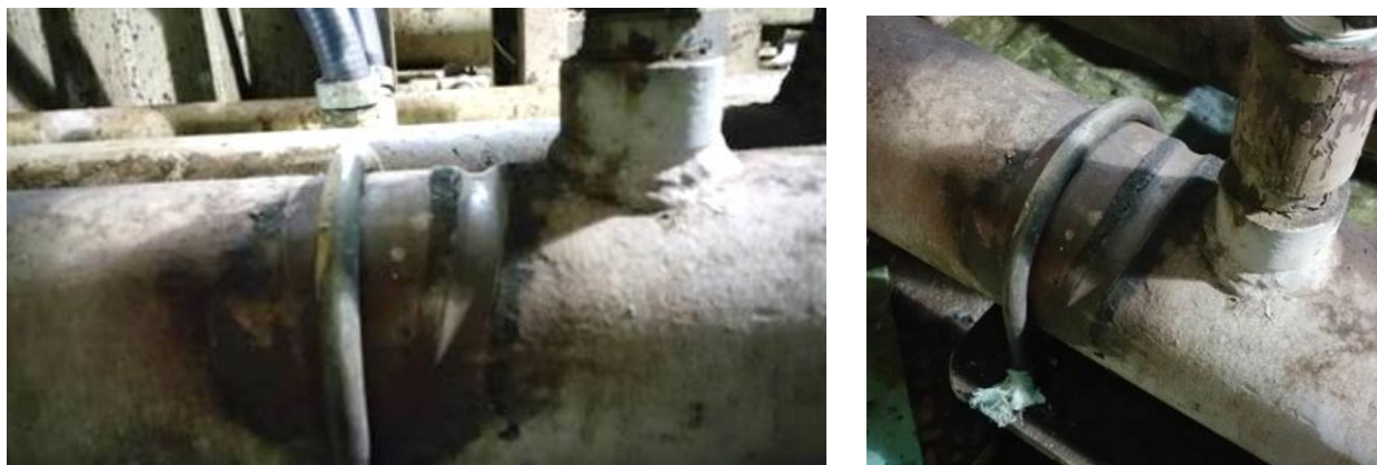
Figure 10. Fretting of U-bolt
