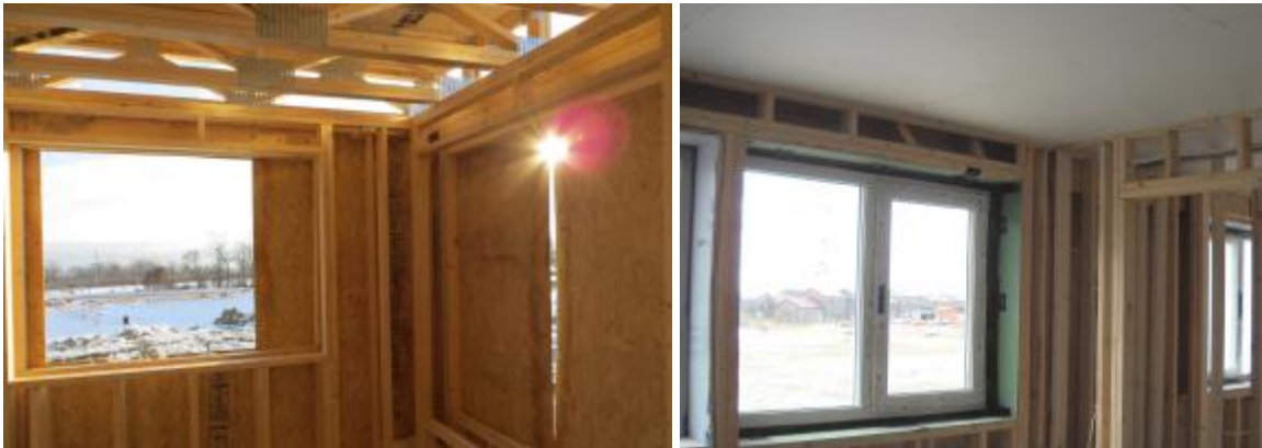
Figure 13. Windows in double walls: (left) a framed window opening and (right) a set window
