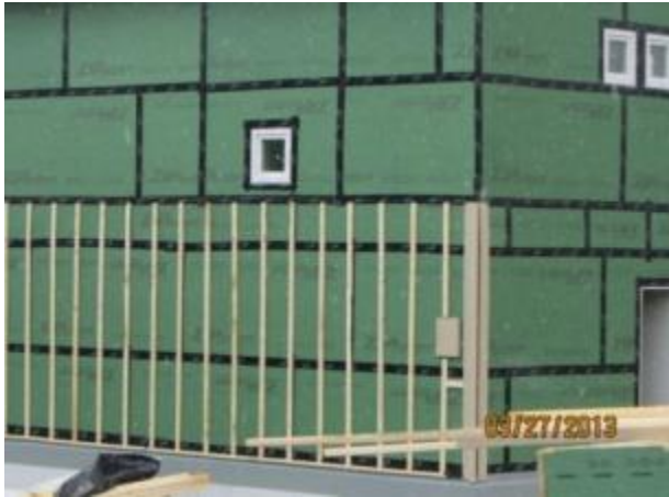
Figure 20. Vertical furring strips create a vent space for horizontal fiber cement siding.
