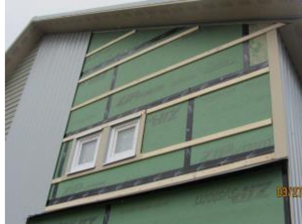
Figure 21. Horizontal furring was used to attach a corrugated metal panel siding that allows vertical draining and venting of the sheathing.
