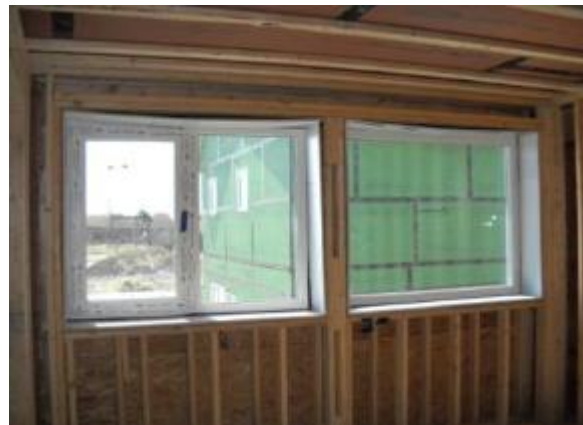
Figure 11. Reduced framing around windows on the interior wall
