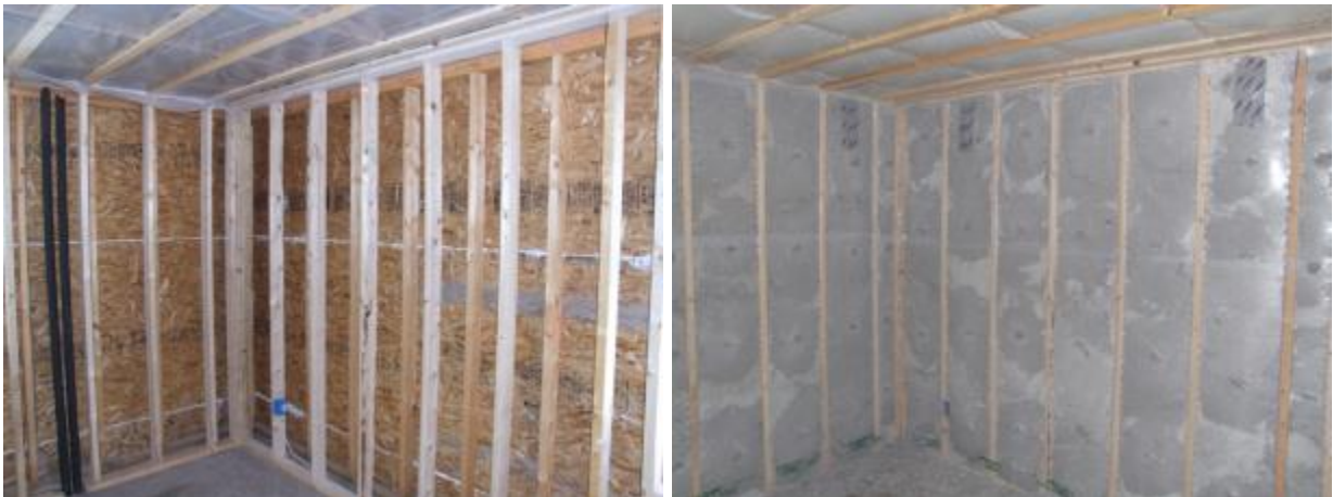
Figure 16. Double wall before and after insulation with dense-blown cellulose
