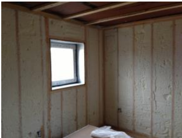
Figure 2. ocSPF in a 12-in. double wall
