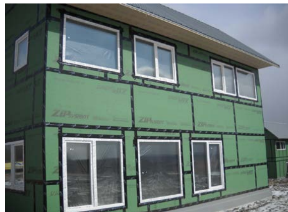
Figure 15. Exterior air barrier with all seams taped
