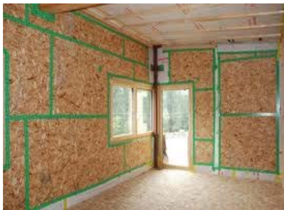
Figure 14. Interior air barrier with all seams taped
