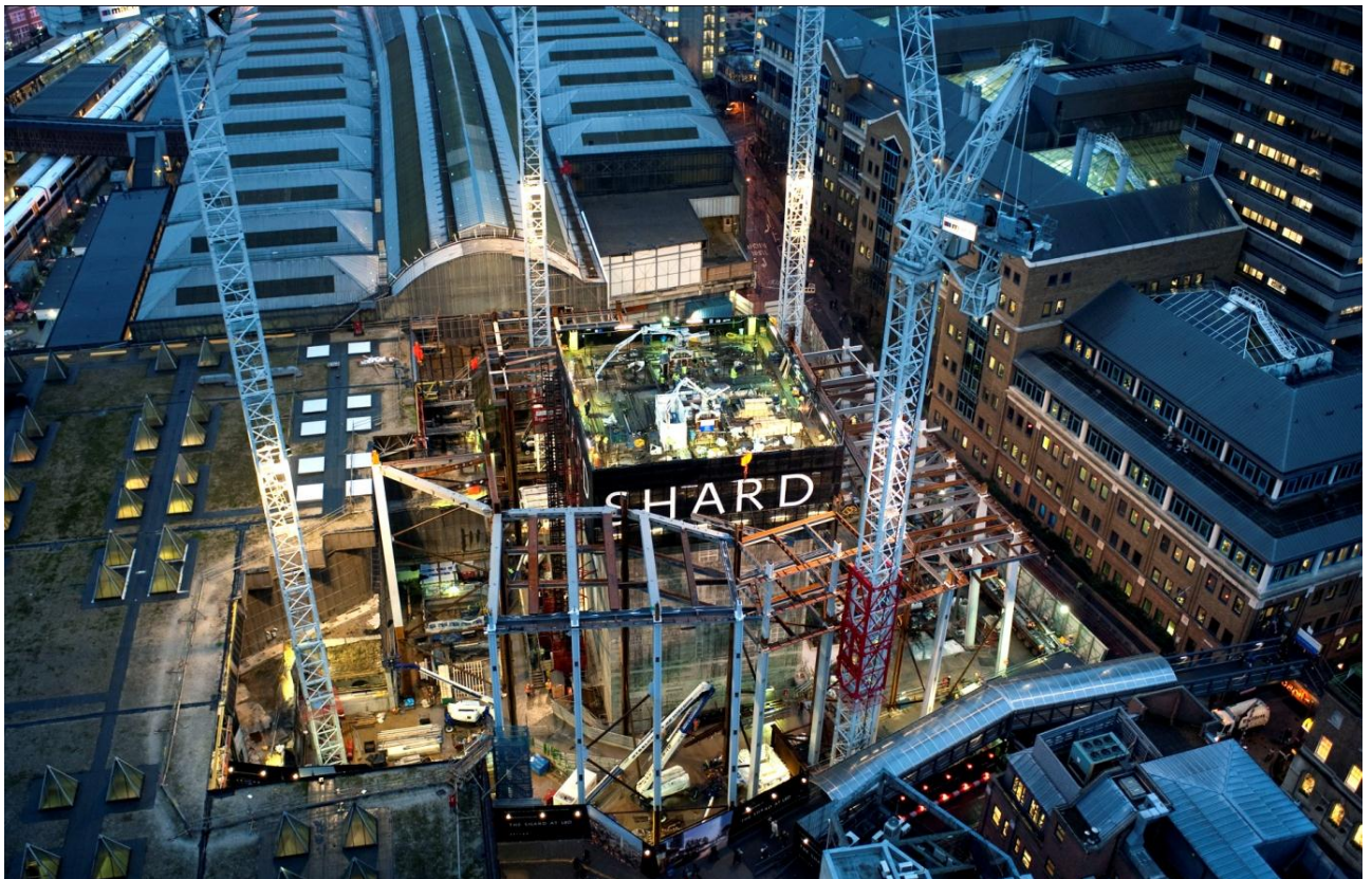
Figure 4– The slipform rising through the steelwork.
