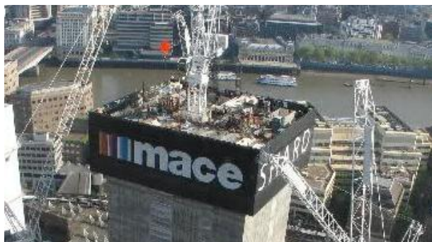
Figure 11 - TC1 within the slipform
