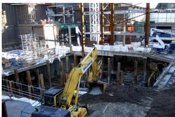
Figure 7 – Excavation to B2. Ground floor ring beam is evident.
