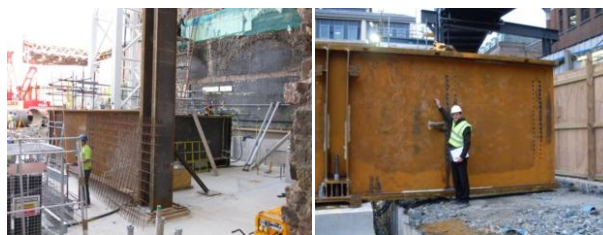
Figure 9 – TC2 and TC5 Crane Bases
