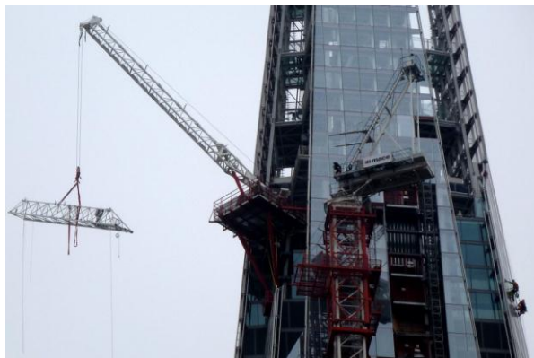
Figure 12 – TC7 Jib Removal
