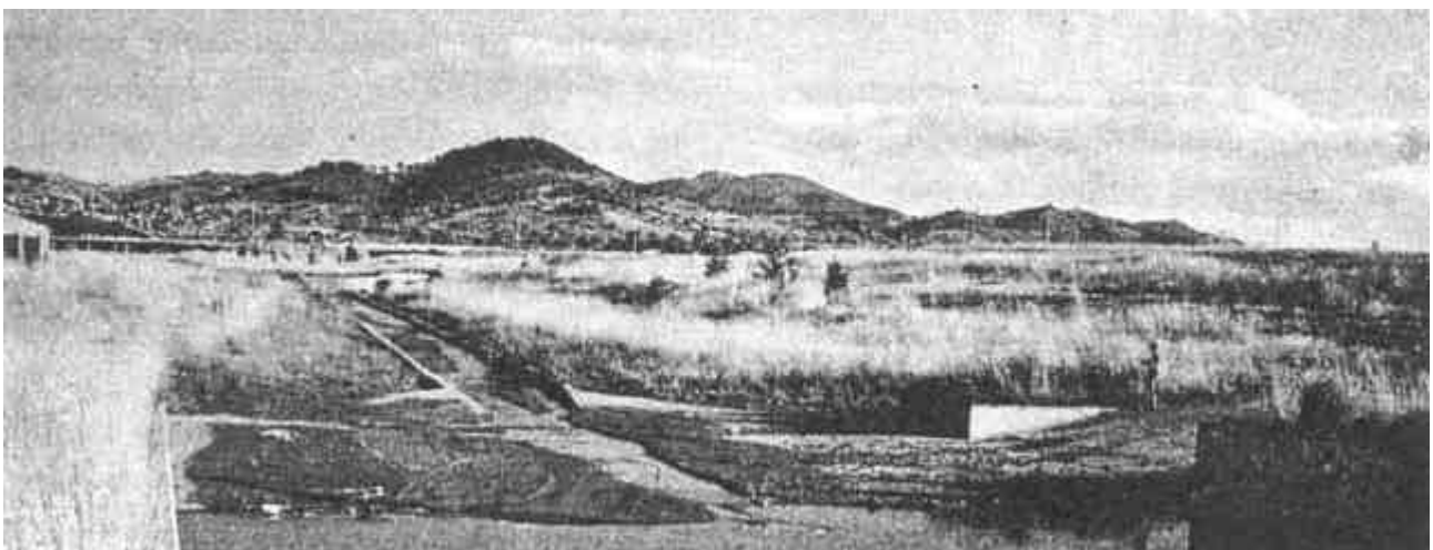
Figure 32. Sediment trap with a sloping concrete ramp to enable easy sediment removal.
