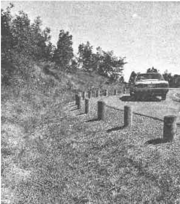
Figure 38. Roadside tabledrain stabilized with grass.
