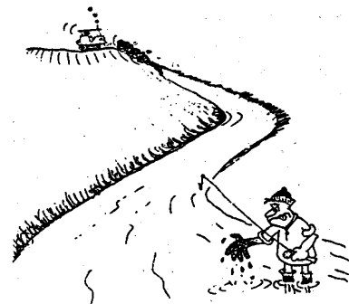
Figure 20. Soil pushed directly into streams results in water pollution. This can usually be avoided by careful planning based on the techniques listed in this booklet.
