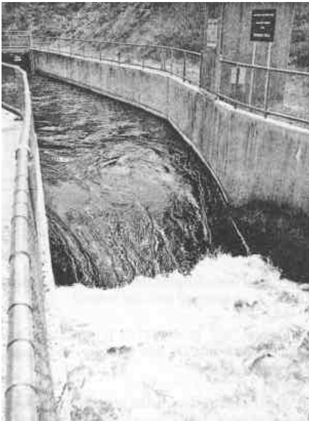
Figure 23. Stilling basin used to dissipate water energy.
