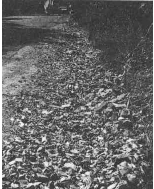
Figure 17. Crushed rocks of about 60 millimetres diameter need to be compacted into a rounded “spoon drain” shape.
