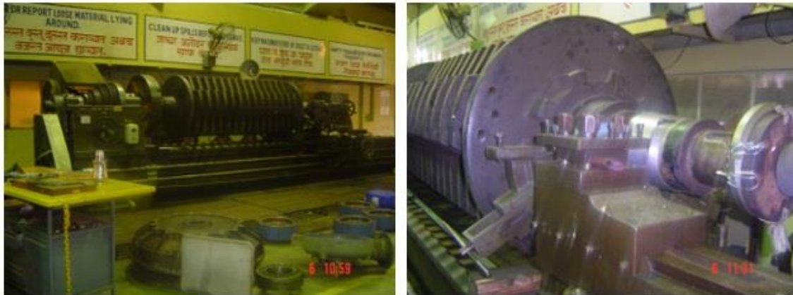
Repair of Granulator Shaft
