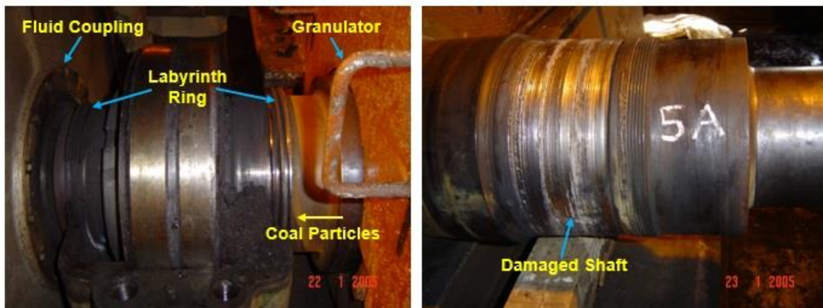
Damage to Granulator Bearing and Shaft
