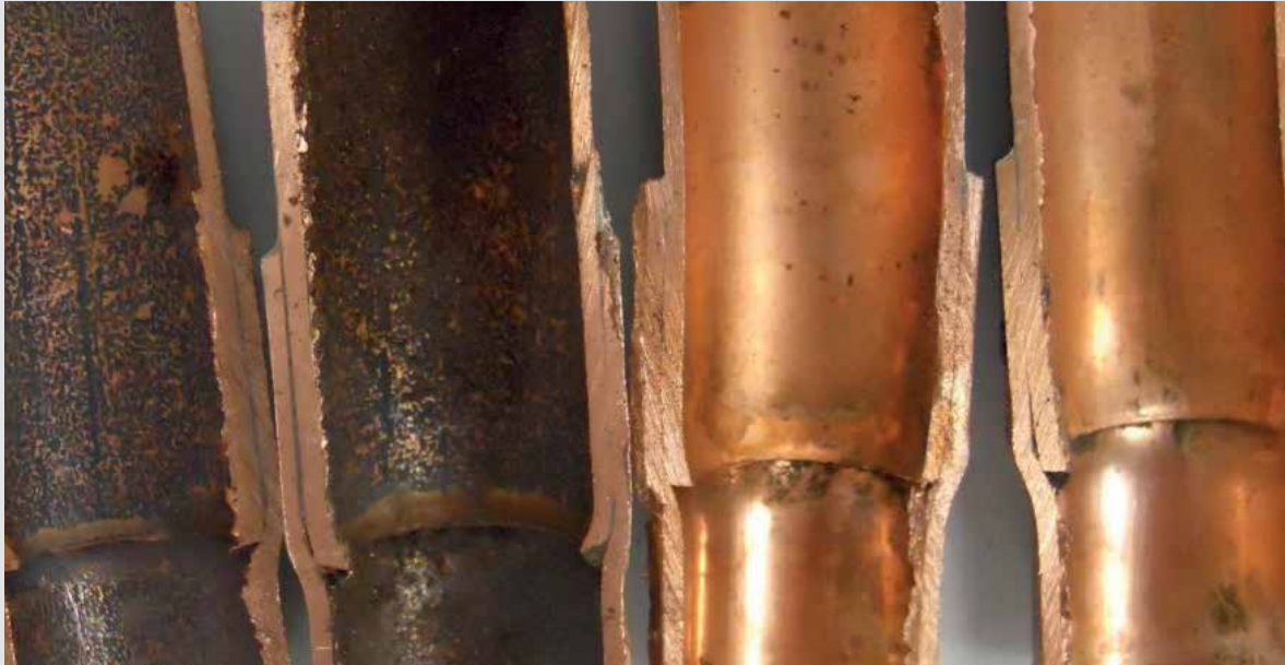
Without nitrogen purge
