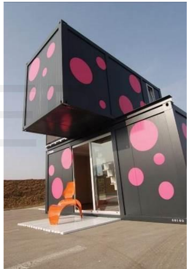
Fig 11: crisscross configuration of 2 containers on top of each other.
