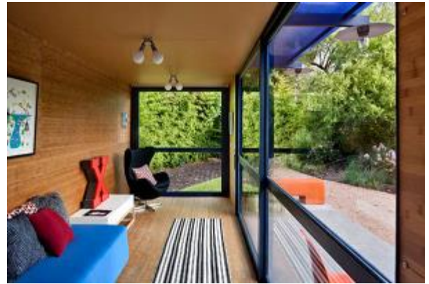
Fig 14: using wood for the internal planes to change the industrial look of the container.
