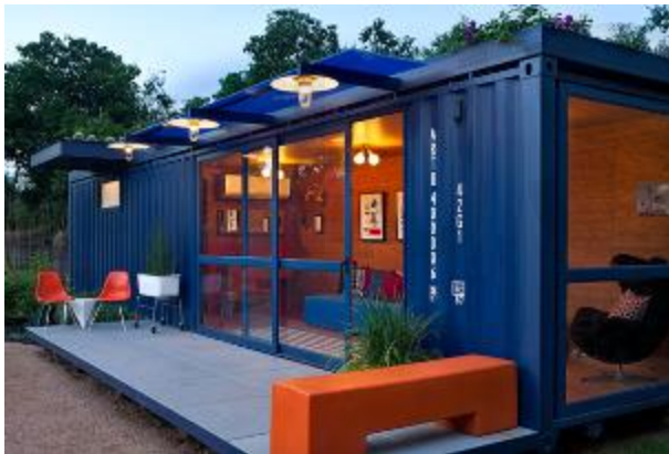
Fig 12: Making some modifications in the vertical planes to create doors and windows.
