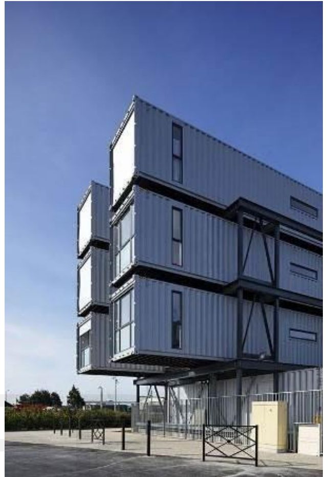
Fig 36: a steel skeleton was constructed to host the containers.
