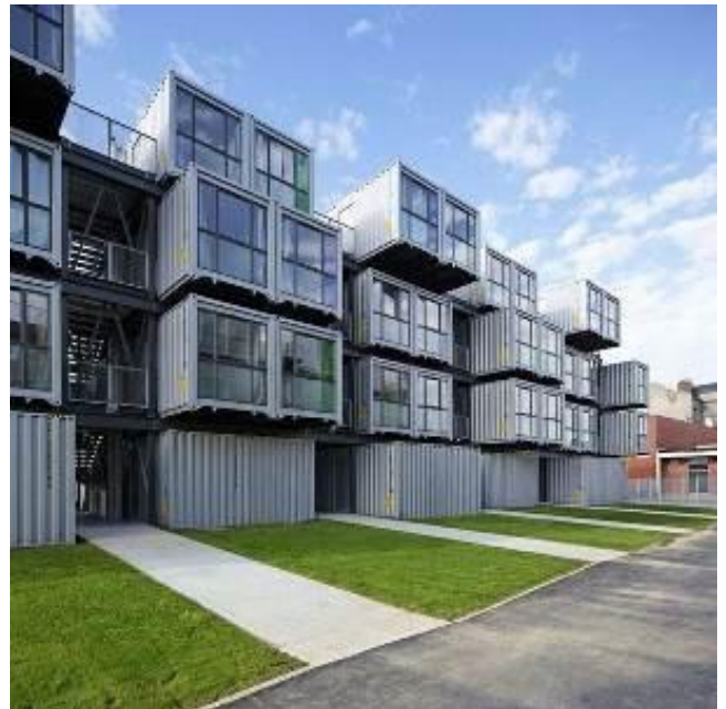
Fig 34: stacking the containers.
