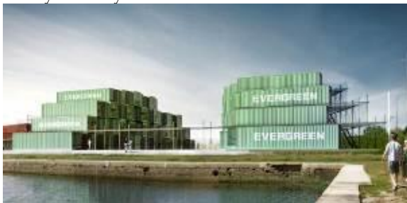
Fig 44: 'Crou' student housing made from 100 recycled shipping containers.
