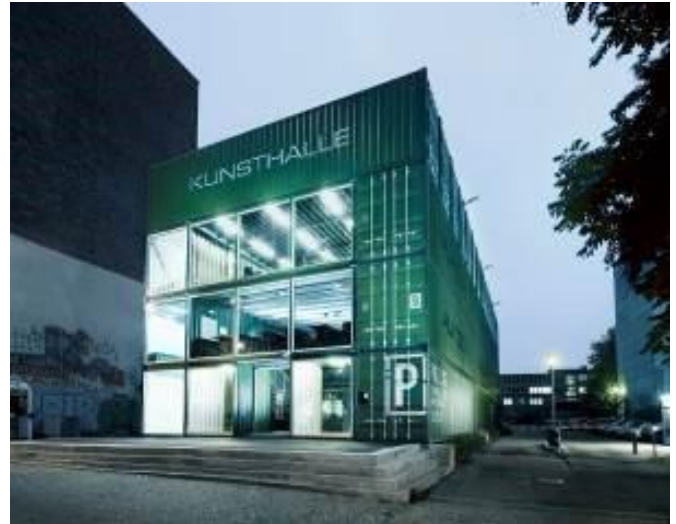
Fig 39: creating a transparent elevation by removing the doors and replacing them with glass panels.
