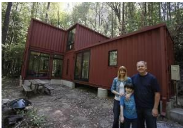
Fig 18: various configurations of staking the containers can lead to various models of residential units.
