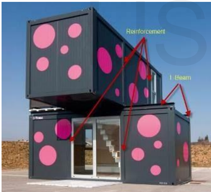
Fig 9: 2 Containers on top of each other
