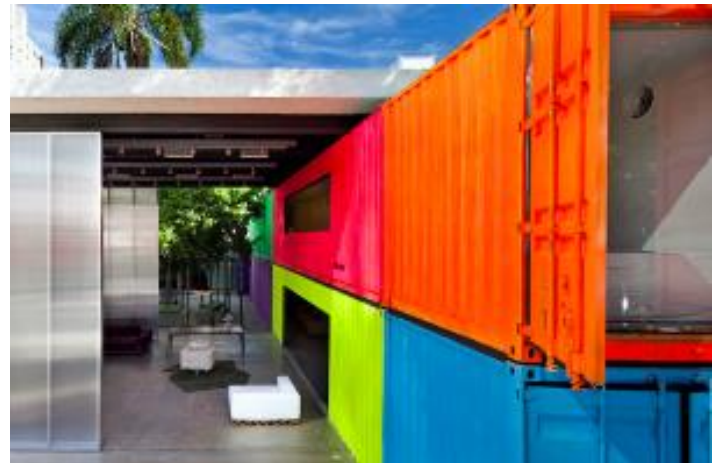
Fig 28: the designer worked on creating dynamic external spaces.
