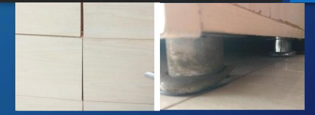
Observe that the drawers are closer at the top than they are at the lower part. Observe also that there are two metal supports on each side as shown in the photograph. We created the support structure in Fusion 360 as shown in the next slide and simulated the loading
