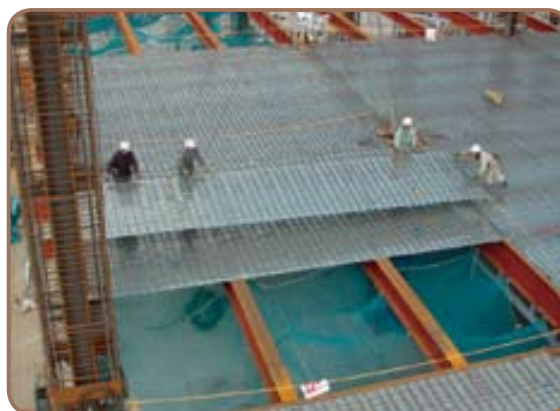
Fab deck floor mold work site
